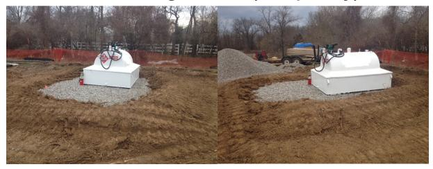
A permit is required for the placement and use of any fuel storage tank exceeding 50 gallons liquid capacity. The tank must be installed, operated and maintained in accordance with the 2024 Edition of the International Fire Code (IFC) Chapter 57.
